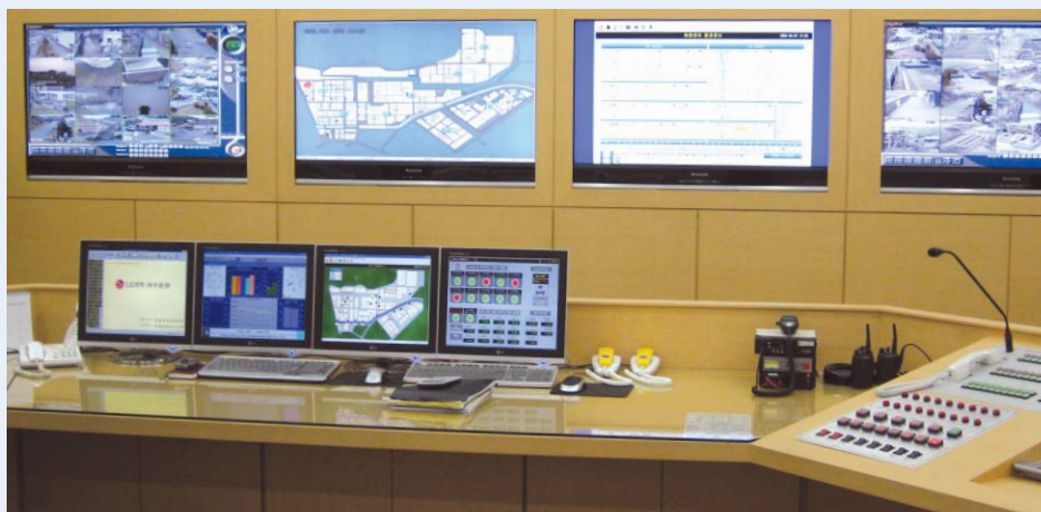
● Emergency Control Center (Yeosu)
