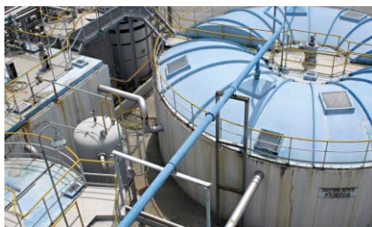
● Wastewater Treatment Plant (Yeosu)
