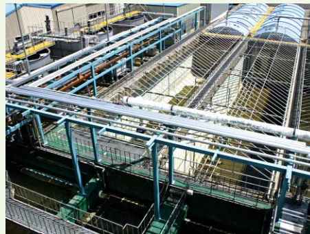
• Wastewater Treatment Plant (Ulsan)
